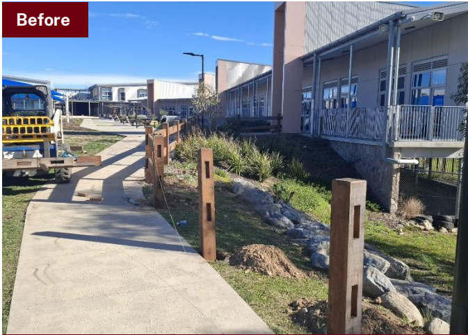
Fencing posts being installed during the school holidays
